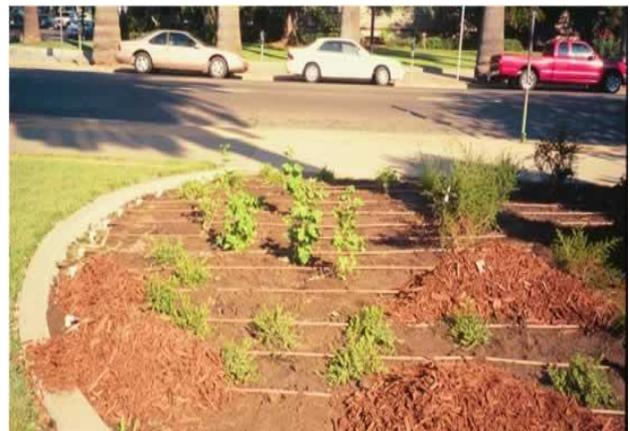
Drip systems can also be installed by converting the existing sprinkler heads.
