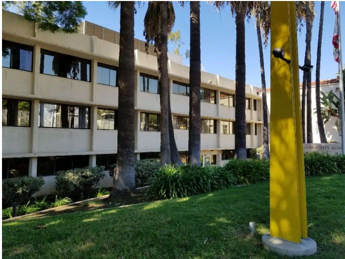
Public Health Building
