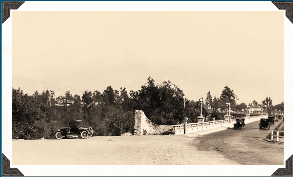
Colorado Street Bridge, circa 1919-1931
