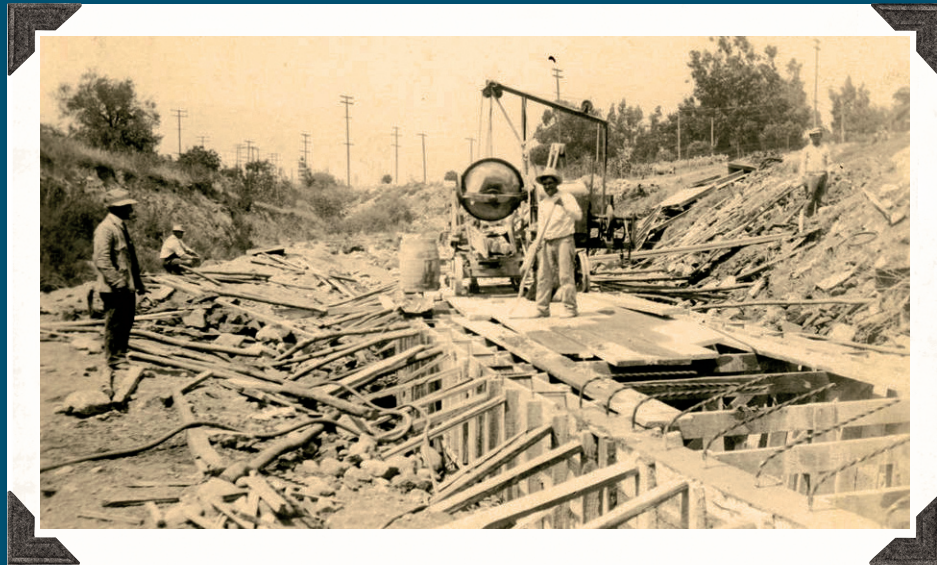
Storm Drain Under Construction, 1916
