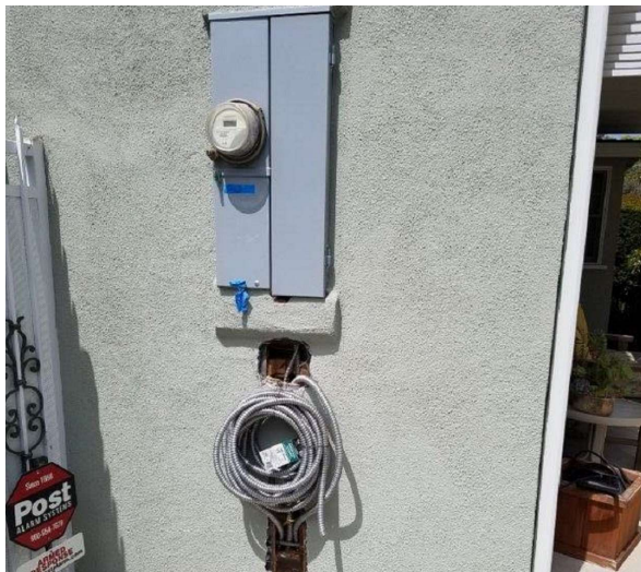
Underground Service Conversion
