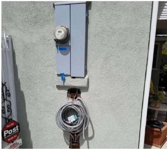
Underground Service Conversion
