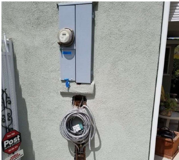
Underground Service Conversion
