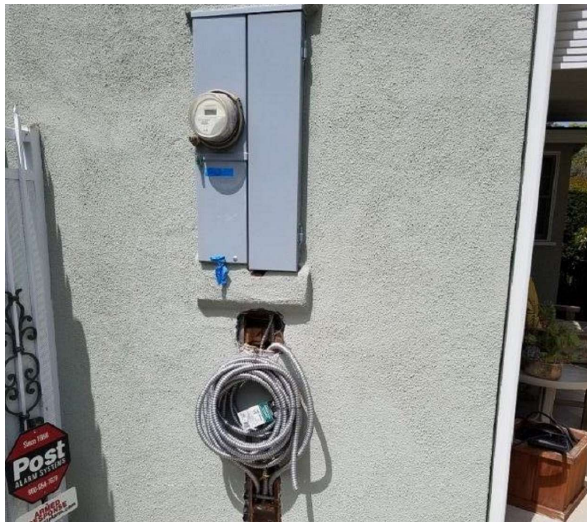
Underground Service Conversion
