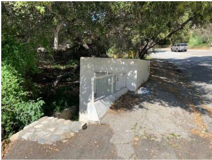
Rosemont Sewer Pump Station
