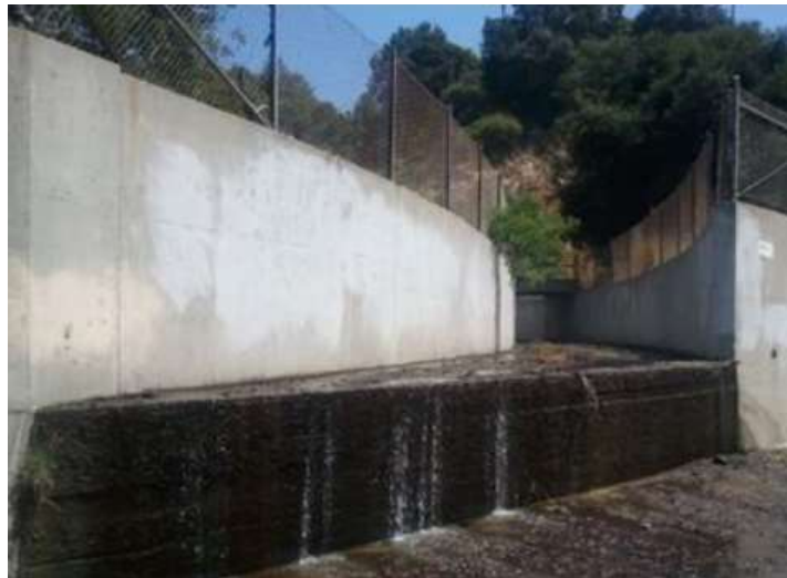
Arroyo Seco Outfall
